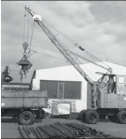
1962: rope-driven S833 with elevated operator cab
